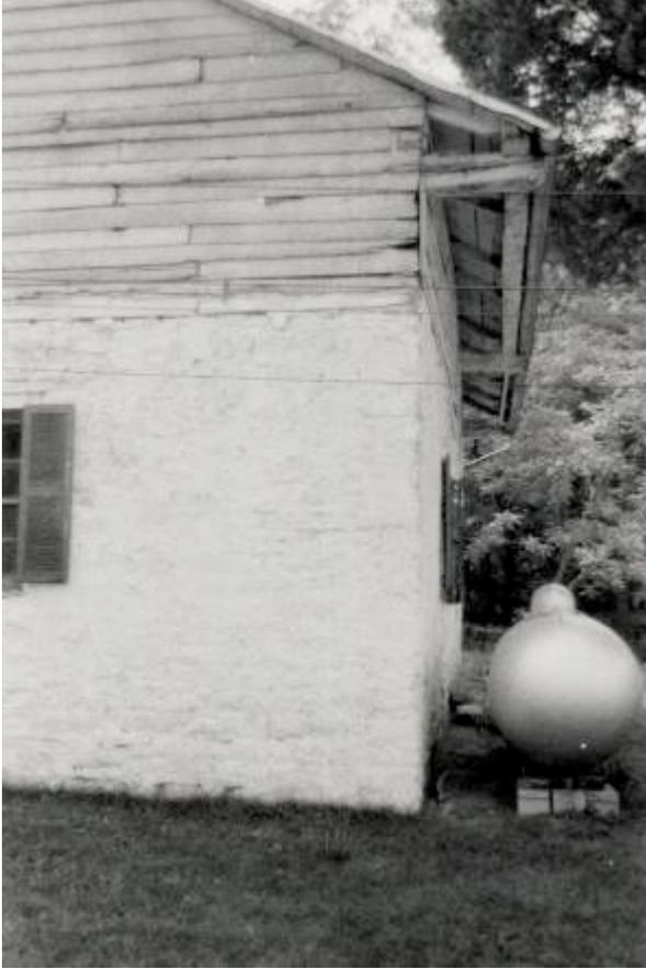
This house is stone on the first floor and has probably four courses of logs resting on the stone to form the upper half story. Unique to this house type is the detail that supports the overhang of the roof. One transverse log at each gable was extended by 4 to 5 feet, sometimes on one façade and sometimes both front and back.
