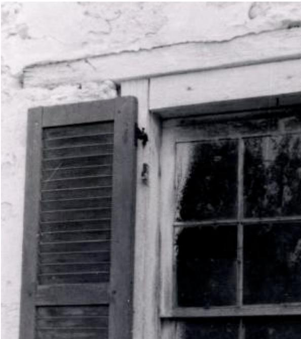
The window frame is of interest because it has evidence of earlier material. The Venetian style shutter is modern, but behind it in the post of the window frame is what is called a pintel. It is a right-angled iron piece driven as a spike into the wood window frame. At the right angle it supports a post that fits into a socket on the shutter. There are two for each shutter and on them the shutter swings open and closed.
